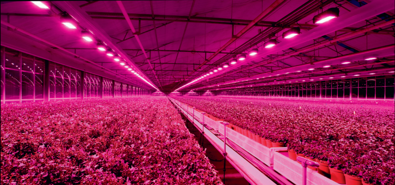
FL300 fixtures covering more than 1.500 m 2 in production unit 11 at PKM.
