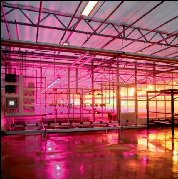
Cell 3 and 4 at the Kold College School for growers. The climate and the LED light are controlled by the LCC 4 climate computer of Senmatic.
